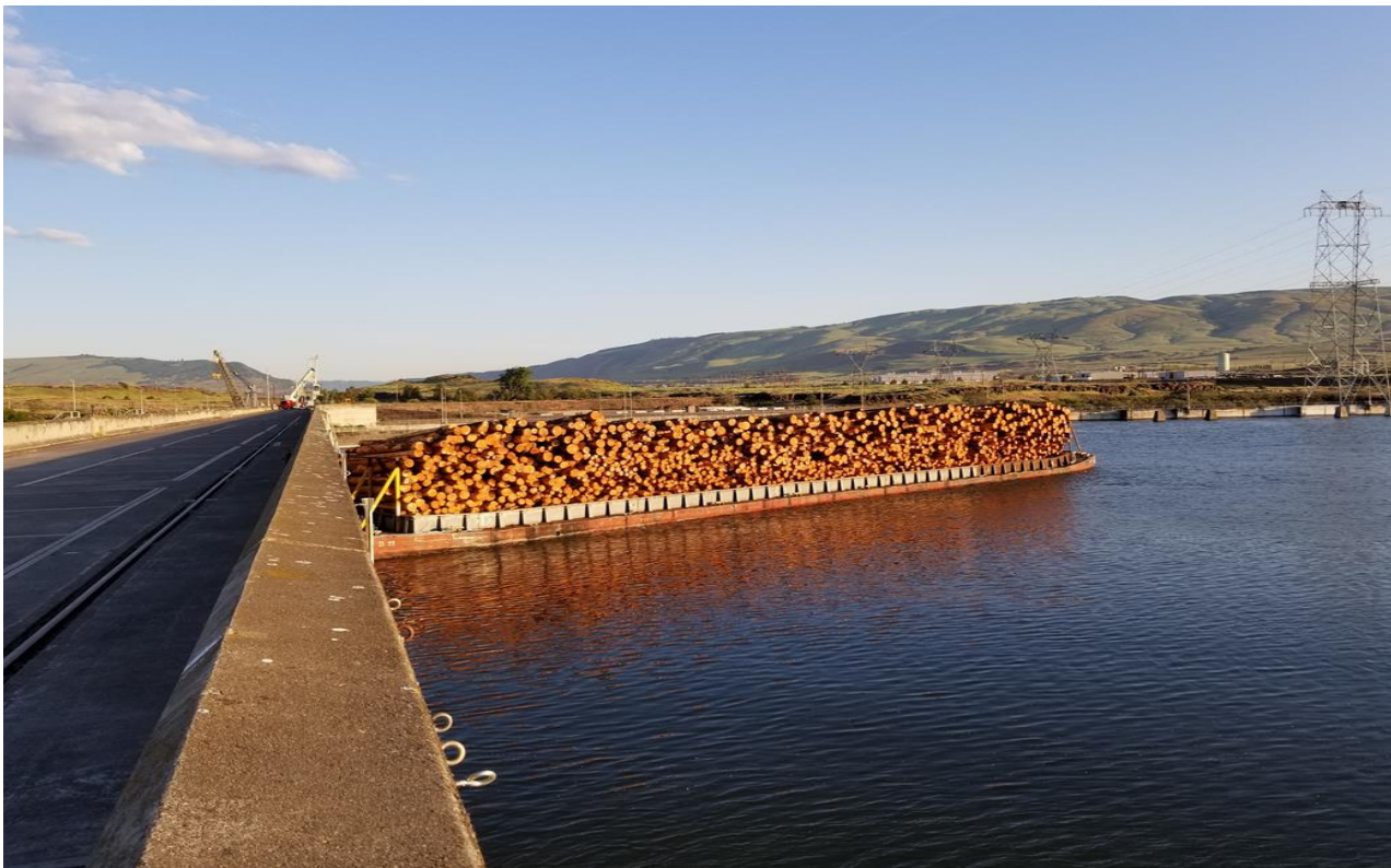
Loose barge tow against spillway May 9 AM. No spill adjustments were needed for removal.
